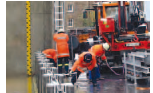
Fire fighters building a flood barrier
