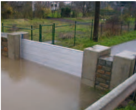
Flood protection barrier protecting an entrance
